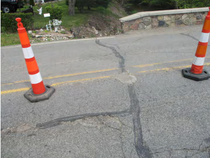
Document Name: 6.JPG Category: Joints Span Number: Comments: East reference line
