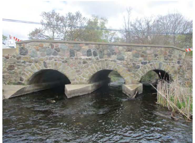
Document Name: 23.JPG Category: Elevation Span Number: Comments: South
