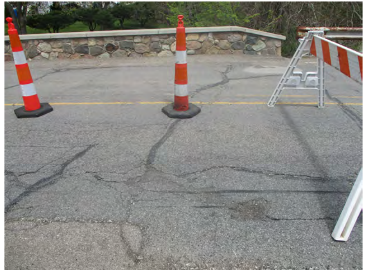
Document Name: 5.JPG Category: Joints Span Number: Comments: West reference line
