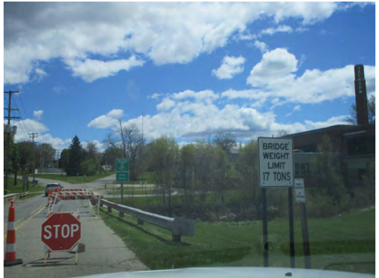
Document Name: 3.JPG Category: Posting Span Number: Comments: West
