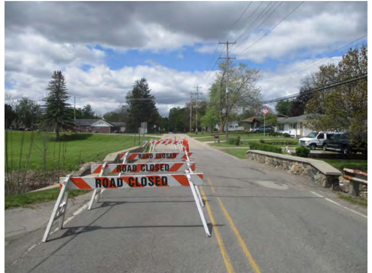
Document Name: 4.JPG Category: Deck Span Number: Comments: Looking west, closed eastbound lane
