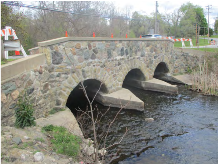
Document Name: 20.JPG Category: Elevation Span Number: Comments: South
