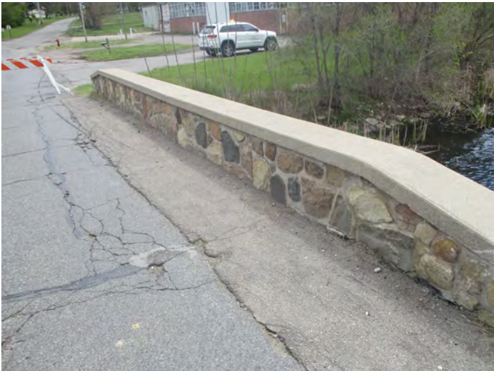
Document Name: 7.JPG Category: Railing Span Number: Comments: South
